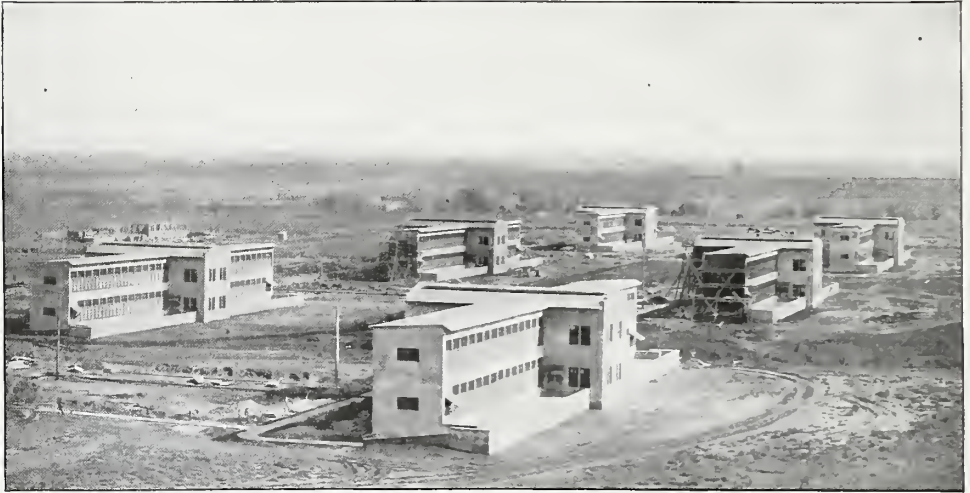
FIG. 113.—Wards (under construction), General Hospital No. 21.
